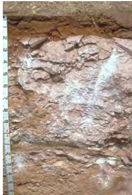
Restrictive calcrete layer at shallow depth (20cm)
